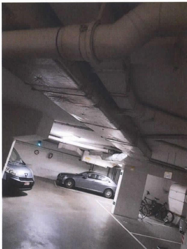
Figure 27: Isolation des gaines de ventilation
