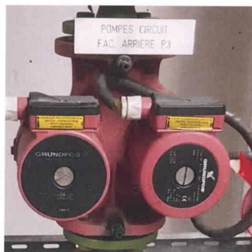
Figure 13: Plaque signalétique P3
