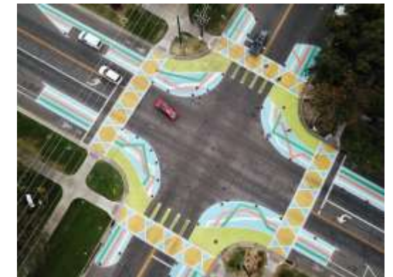
Intersection remodeled for biking
